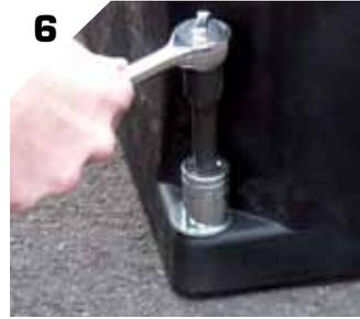
6 Tighten the anchors to 22.0Nm torque for concrete. Tightening will fan out the bolt sheath in the hole holding it secure.
