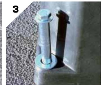
3 Add the large washers to the anchors. Then place the anchors, with washers through the moulded holes into the holes in the ground.
