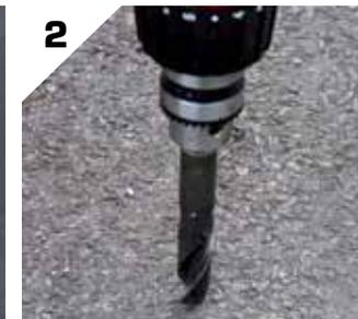
2 Using a 16mm diameter masonry drill bit, drill 4 holes to a depth of 110mm and remove debris from holes.
