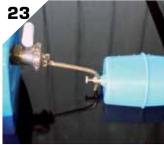
23 Placing the float at the bottom of the arm, sets the lowest possible water level, and at the top of the arm, the highest water level.
