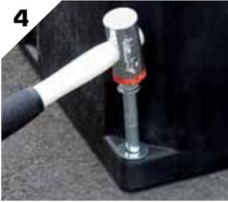
4 The anchors should be a tight fit and will need to be driven home with a mallet.
