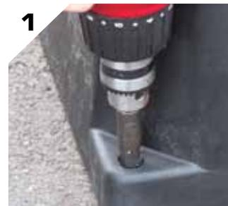
1 Locate the 4 ground fixing holes at the 4 corners of the trough. Place the drill through the holes and spot drill the locations.
