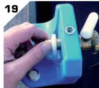
19 Remove the ballcock cover to gain access to the float valve. Loosen the nut so that it is 3-5mm from the support wall.
