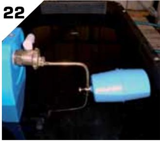
22 The plastic float valve height can be adjusted to set the water level in the trough.
