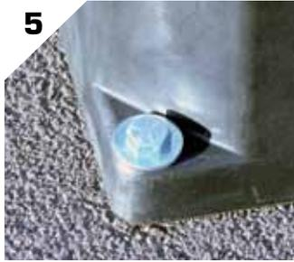
5 Ensure the anchors have been driven all the way home and there is no gap between the washer and the moulding.
